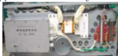
Figure5 Battery management system management to each cell, and on-line forecast the remainder electricity (SOC) of system to ensure the battery life and high efficiency applications.
