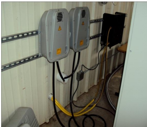
Figure 20 Capacitor Boxes used to Tune the Circuit
