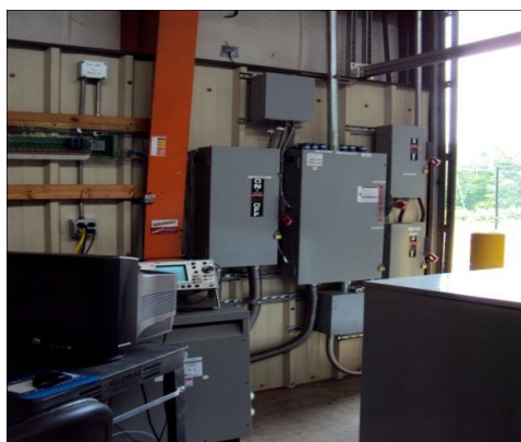
Figure 16 Switch Gear, Voltage Transformer and Data Acquisition System
