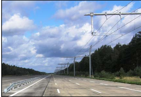
Figure 3 – Overhead contact line, roadway and protective equipment
