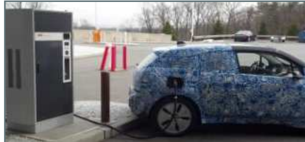
BMW of NA – Woodcliff Lake, NJ BMW i3 operating an ABB DC 50 kW unit
