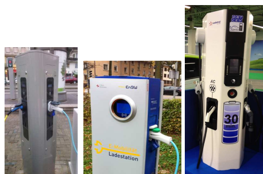
Figure 2: CROME interoperable public charging stations: 2 x “mode 3” (type 2 and 3) in Strasbourg (left), 2 x “mode 3” (type 2 and 3) in Kehl (middle), and 43 kW DC fast charging mode 4 in France (right).
