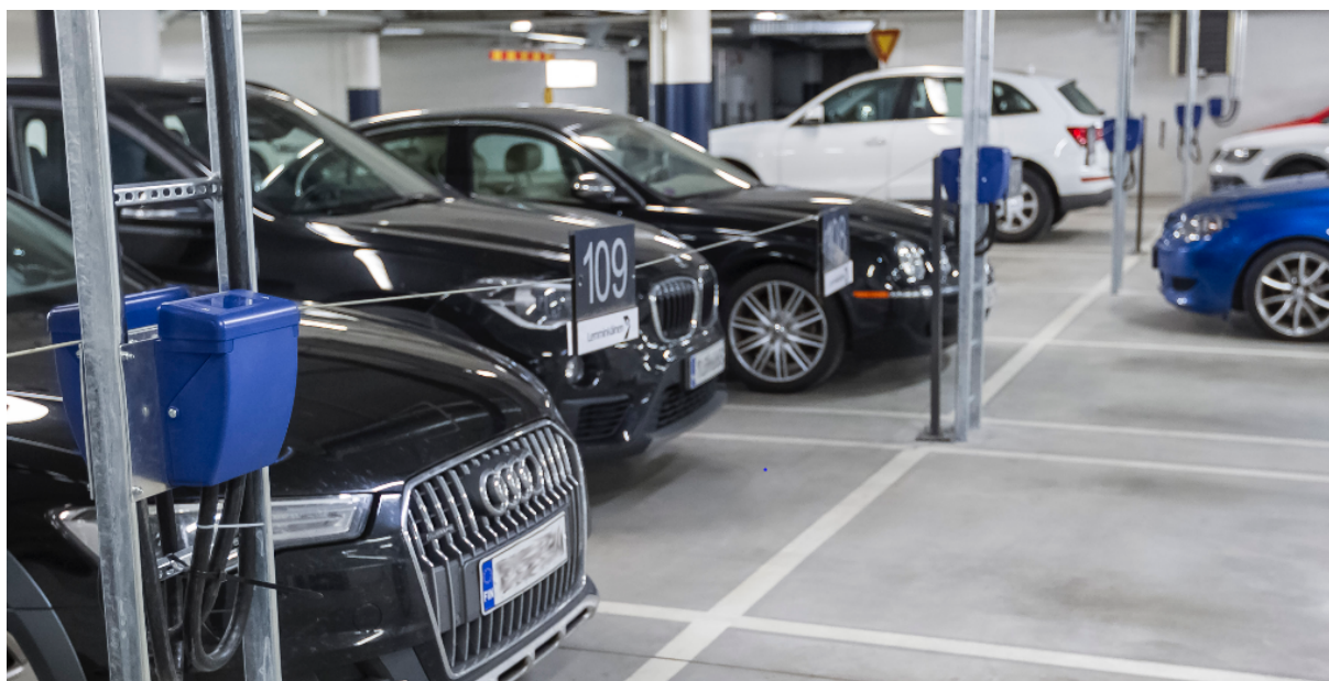
Figure 2: All parking spaces equipped with Quick Connector cabling; one connector for every two parking spaces, offering up to 44 kW.
