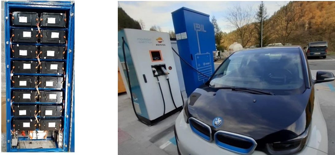
Figure 5: (left) 75 kWh BESS during the assembly process (right) Charge point and BESS in Repsol's service station in Tolosa, Spain.
